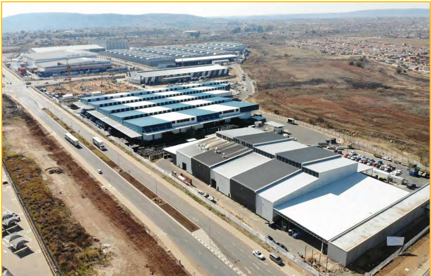
Tshwane Automotive Special Economic Zone construction update, with Coega as the Infrastructure Implementing Agent of Choice: A Case Study for South Africa's Infrastructure Development Excellence.
