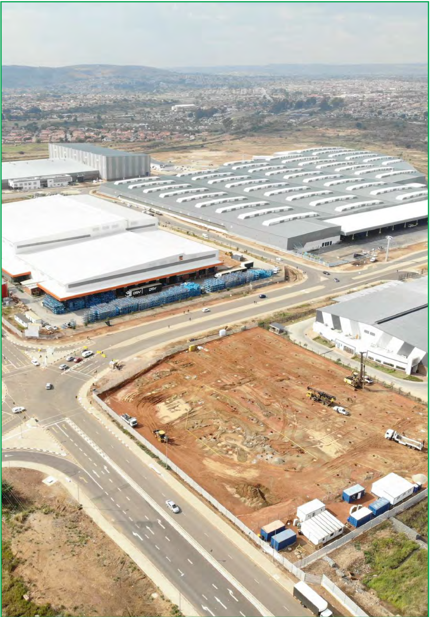
Tshwane Automotive SEZ construction site.
