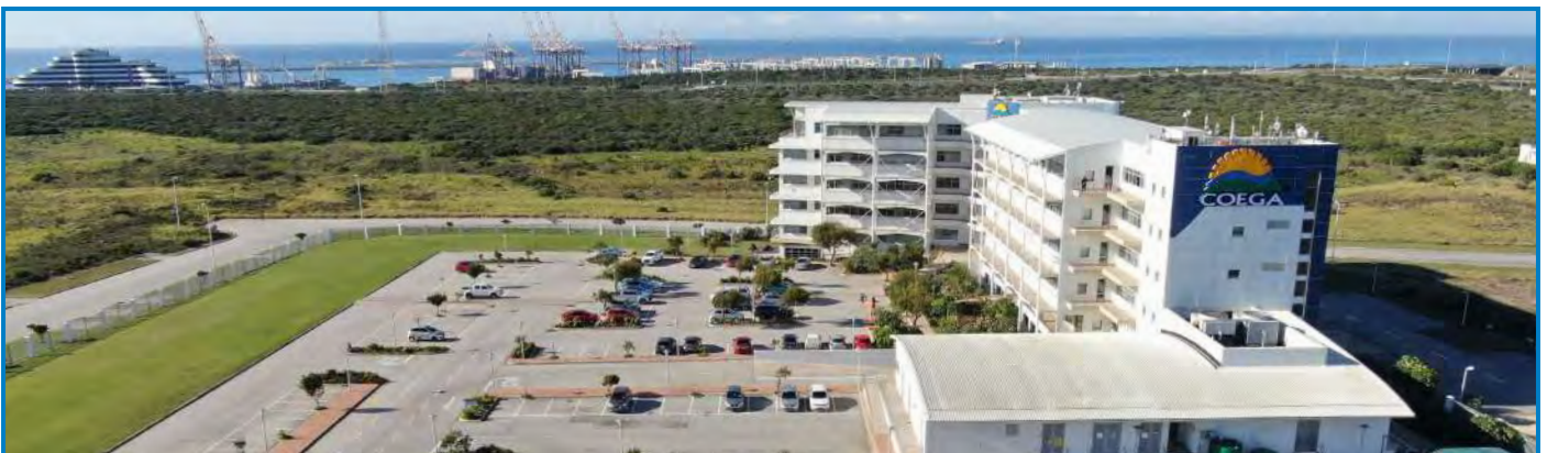
The Head Office of the Coega Development Corporation, with the Port of Ngqura and TNPA Office in the background.
