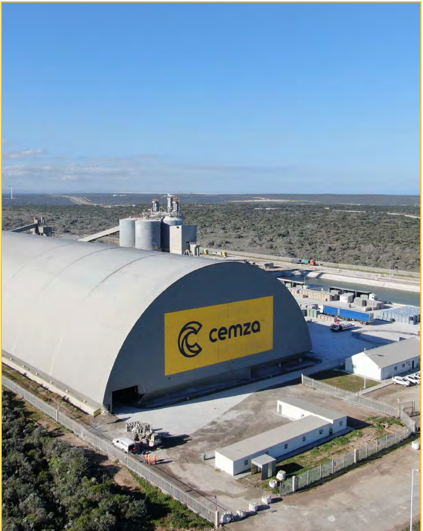
CEMZA located in Zone 5 of the Coega Special Economic Zone, Gqeberha.
