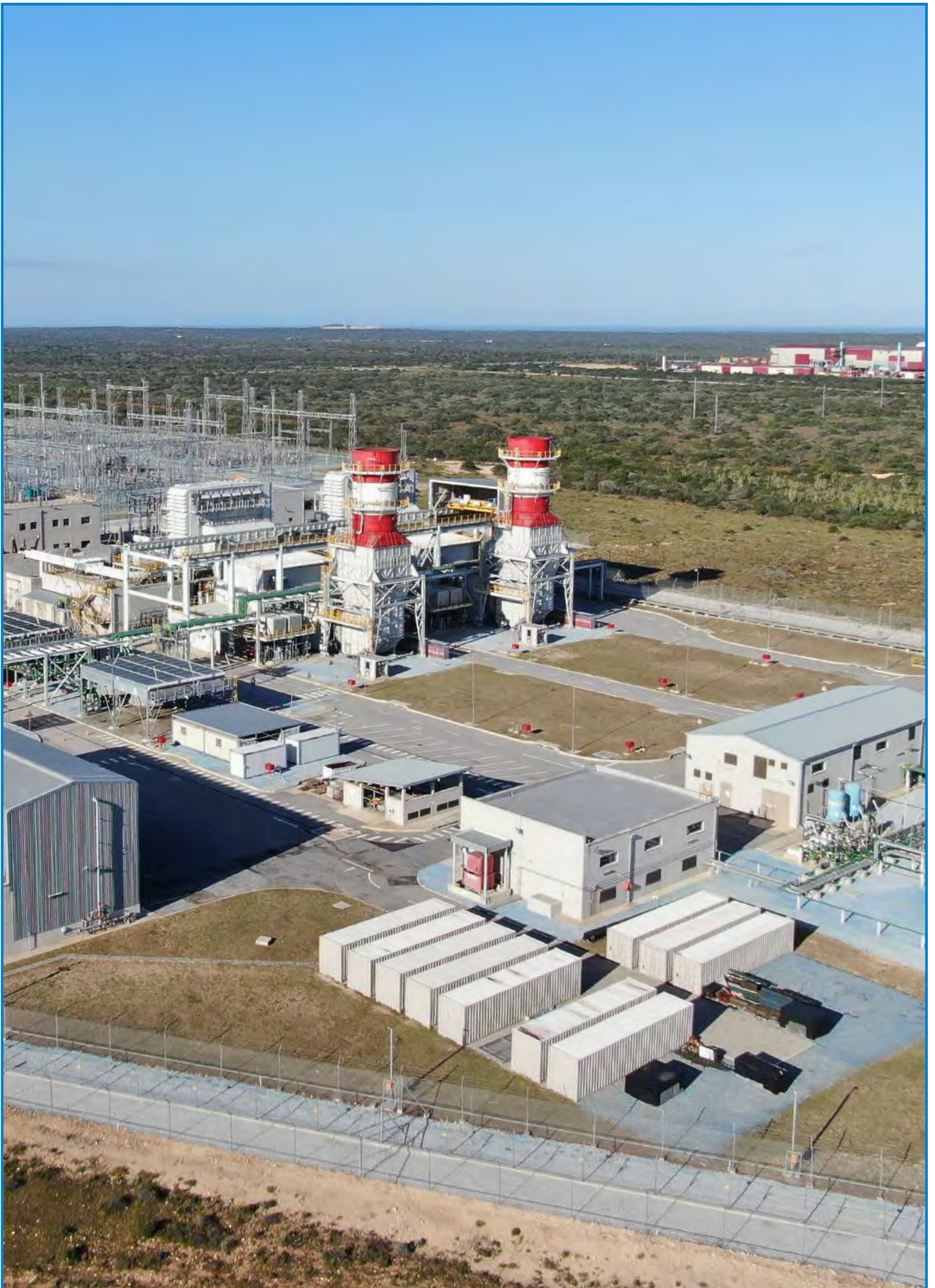
The DEDISA Peaking Power Plant in Zone 13, Coega SEZ.
